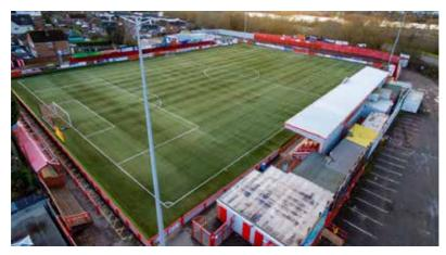
Since the start of last season there have been some big changes at the Lamb which you can't help but spot. The 9 ageing and second hand floodlight columns have been replaced by 4 brand new state of the art LED floodlight towers. The lights are brighter and cheaper to run, and with the facility to dim them, they are suitable for use in a number of different situations.
